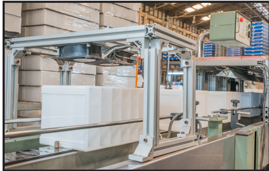
T-Slotted aluminum rail structure holding fans above a conveyor
