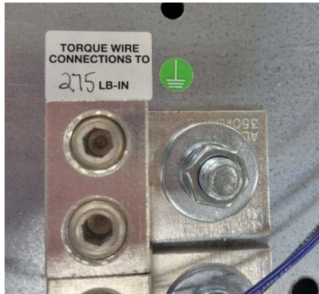
Figure 1: New Connection Lug with Updated Torque Specification
