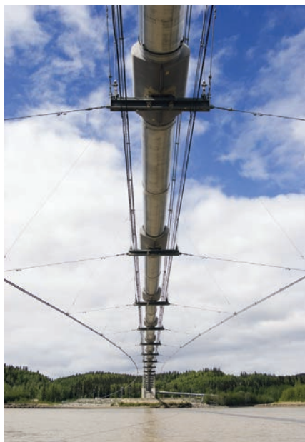
Image 1. Early data acquisition systems were often associated with widely dispersed assets like this oil and gas pipeline.
