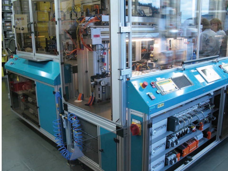
Figure 3: This production cell uses multi-function safety relays to simplify the safety system, cut its cost, and add to its flexibility.
