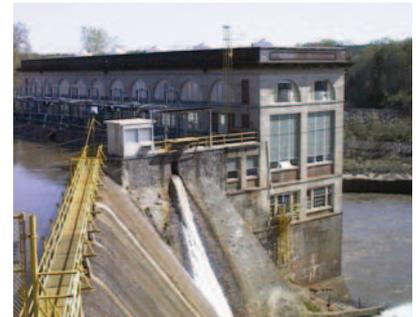
The plant includes an 8-gate dam feeding a canal that channels the water flow to the powerhouse. The powerhouse contains five turbine generators with a combined power capacity of over 17 MW. The dam and turbine control system receives data from power, flow, and level sensing devices to perform monitoring and control of the dam, generators, and associated equipment.
