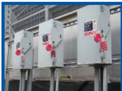
Disconnects with provision for adding lock
