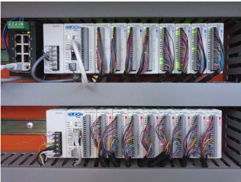
Figure 4: CLICK PLC racks Two racks of AutomationDirect Click PLC hardware are used to monitor safety systems and control train sequencing, brake systems and the air compressor.
