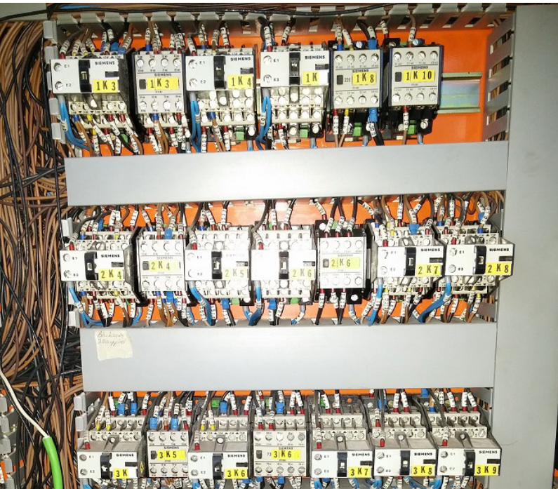
Figure 2: Relays There were several control panels full of hardwired relays and accompanying wiring, causing intermittent problems which were difficult to diagnose.
