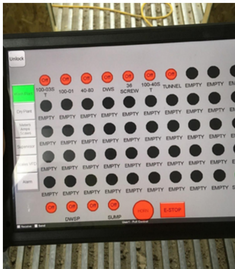
Figure 5: HMI Aids Operators
