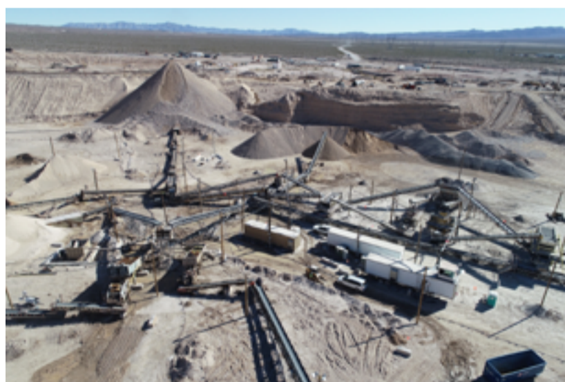
Figure 1: CTC Crushing Processes Overview The surface mine at the top of the photo feeds CTC Crushing's dry processes. The wet process at the bottom left of the photo feeds washed final product to the bulk storage piles, which are not shown.
