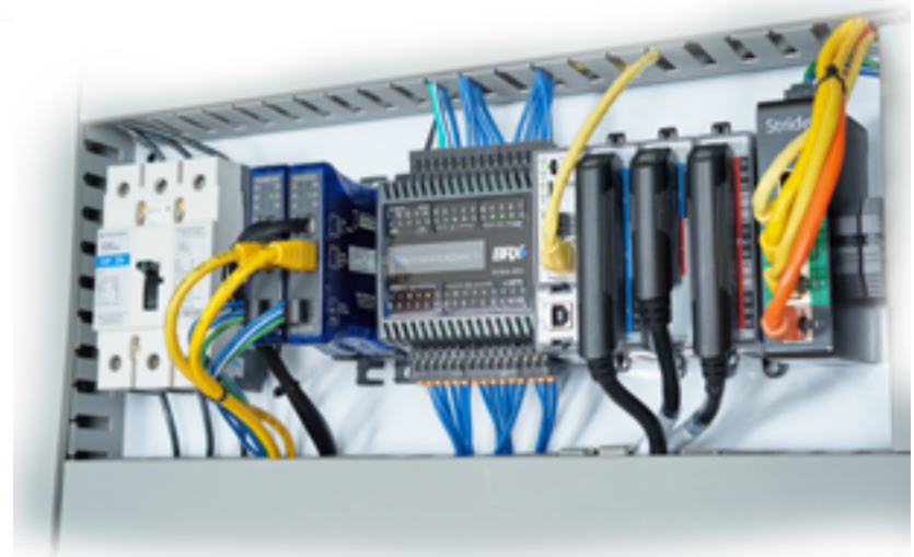
Figure 2: VPN cabinet. By only providing the functionality needed for IIoT connectivity, this AutomationDirect StrideLinx VPN router, installed on the far right of the DIN rail and connected to the PLC, simplifies implementation and use.
