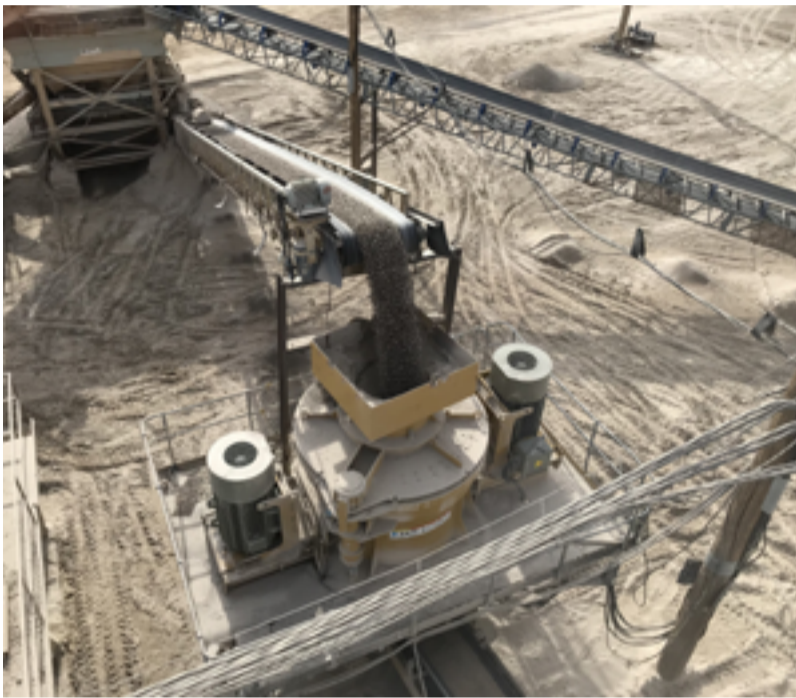
Figure 2: Vertical Shaft Impact Crusher The dry process vertical shaft impact crusher uses twin 400 hp motors to crush 1.5-inch rock to 1/8-inch minus sand that is fed to the wet plant.
