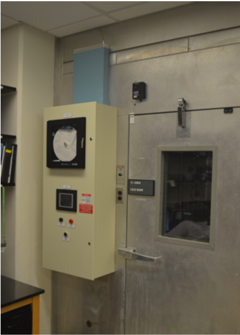
Figure 3: (courtesy of Affinity Energy) Affinity Energy replaced the obsolete controller with an AutomationDirect PLC and HMI due to the open, precise control capabilities and ease of use of these components.
