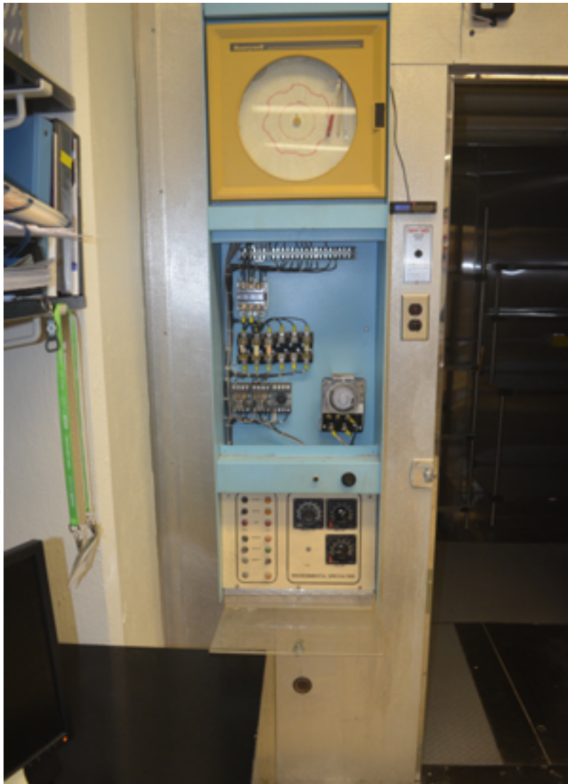
Figure 2: (courtesy of Affinity Energy) The original chamber control system was more than 20-years old and difficult to support, and an upgrade by the original manufacturer would be have been too expensive.
