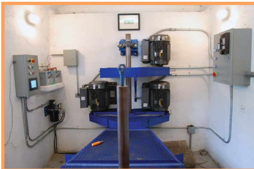
Figure 3: Turbine uses pulleys and belt drives to operate three electric motors.
