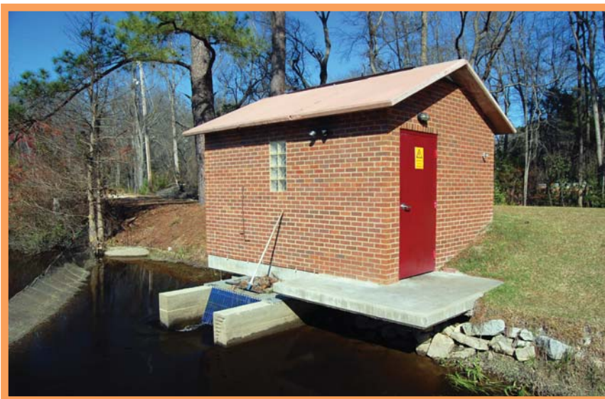
Figure 1: Micro hydroelectric plant
