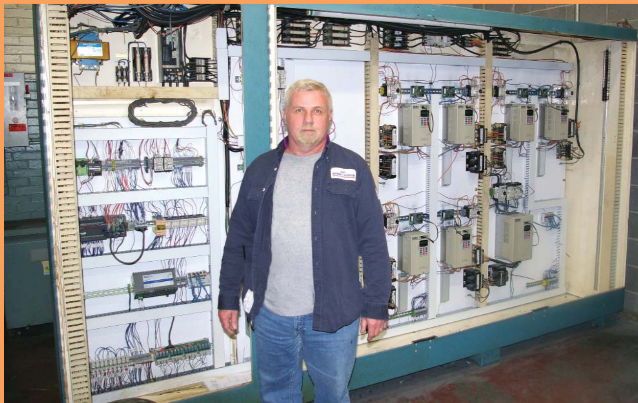
Figure 3, Jonathan Payton stands in front of the new finishing line control cabinet which includes a DL260 Direct Logic PLC, 8 Durapulse variable frequency drives, and all the associated control equipment. The entire design including software was installed during their 3-week shutdown.
