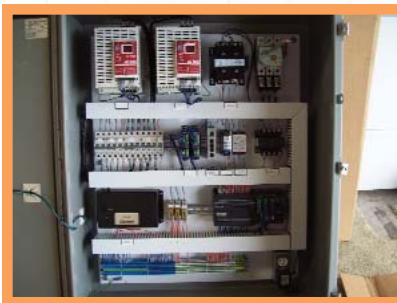
Figure 3, This is a picture of the control enclosure just after completion. It is a simple system using an O6 PLC with various analog functions, and Ethernet for the touch screen, and for future Internet communications. The small black box in the lower left corner is a phone dialer for alarms and system status. Internet is not available in the area.
