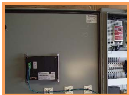
Figure 4, This is another view of the enclosure showing the 6-inch C-more touch screen. The next system will use a larger screen.
