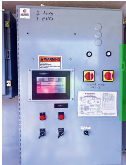
Figure 2: A current-generation AutomationDirect C-more touchscreen HMI was readily retrofitted into the existing control panels, and it was easily configured to replicate the existing functionality and provide new capabilities.
