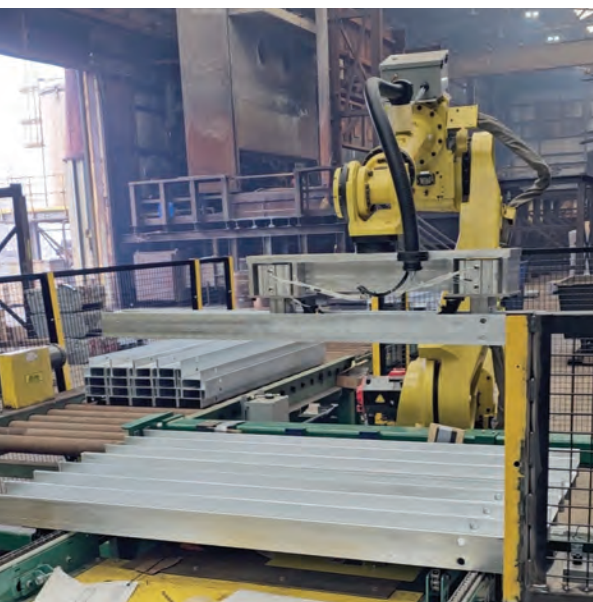
Figure 4: The finished system: PLC-based coordination enables the robot to take newly galvanized posts from the infeed conveyor to be stacked neatly in bundles of 50 before sending them to the forklift staging area.
