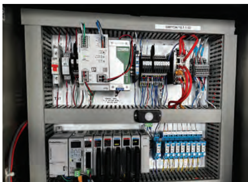
● Figure 3: PLC enclosures include equipment such as switches, breakers, power supplies, the PLC, and even a motion sensor for simulating panel intrusion alarms. The wiring in the test lab BRX PLC cabinet is slightly messy by design to make troubleshooting as realistic as possible.
