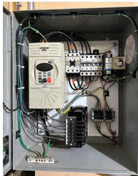
● Figure 2: AutomationDirect VFDs (a GS2 in 2007, and a GS23 in 2025) have provided easy-to-use stage control for the TLP team, and a practical upgrade path away from a problematic hydraulic system. The 2025 upgrade eliminates the ongoing need for three-phase power.
