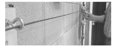
11a. Tension the system by holding the hexagon thimble whilst turning the switch eyebolt
