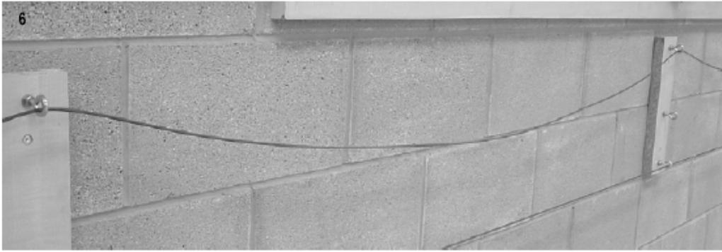
7a. Unscrew the eyehook from the Hexagon shaped Thimble and re-fit the eyehook by 3 turns of the thimble to ensure that the eyehook is secure. Leave the maximum thread possible for later adjustment of the rope tension.
