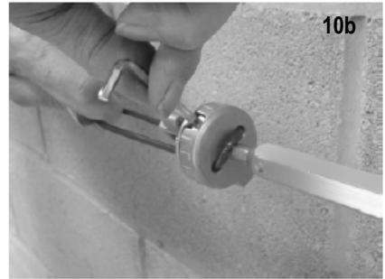
11a. Tension the system by holding the hexagon thimble whilst turning the switch eyebolt
