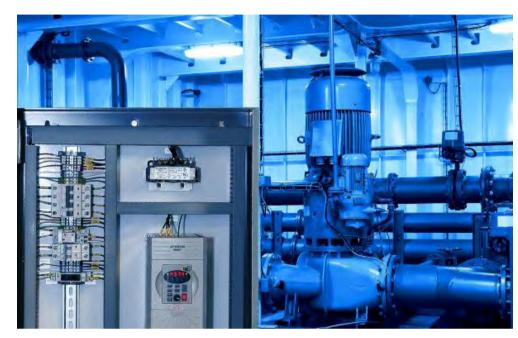
Note that VFDs commonly carry different ratings for use in either CT or VT applications, so the specifier must take care when selecting the drive. If unsure of the application type, choosing the CT rating is the more conservative design approach, and will provide adequate power for either CT or VT applications.
