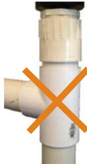
Avoid the use of a tee within the stand pipe. A tee can create false signals which will interfere with the sensor's performance.
